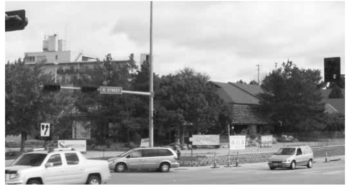
Unightly motel to be demolished.
