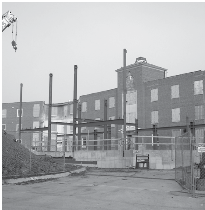
South (Main) Entrance bracing for transformation.
