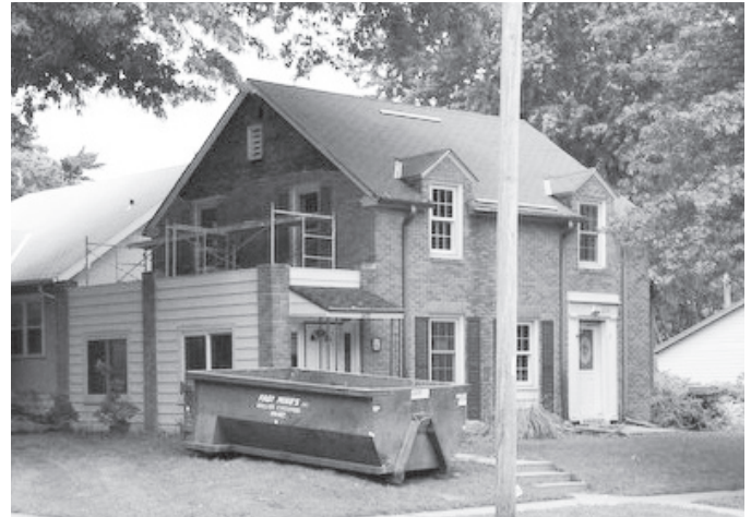
Home remodel begins at 635 S. 36th St.
