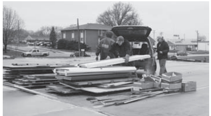
Large stack of construction material was re-cycled.
