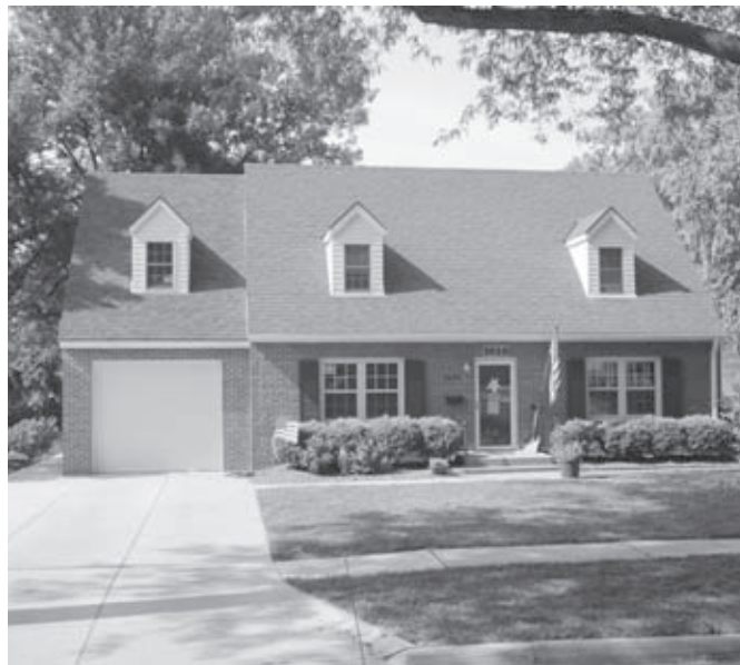
Outside view in July.
