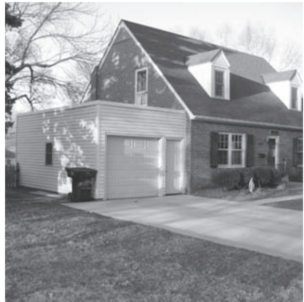
View of home before demo of garage.
