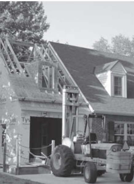
Construction progress in spring.
