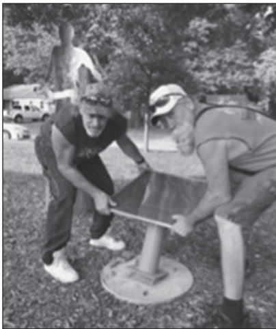
Barry Fox and Rich Hamby of Lincoln Parks and Recreation re-install the repaired pedestal
